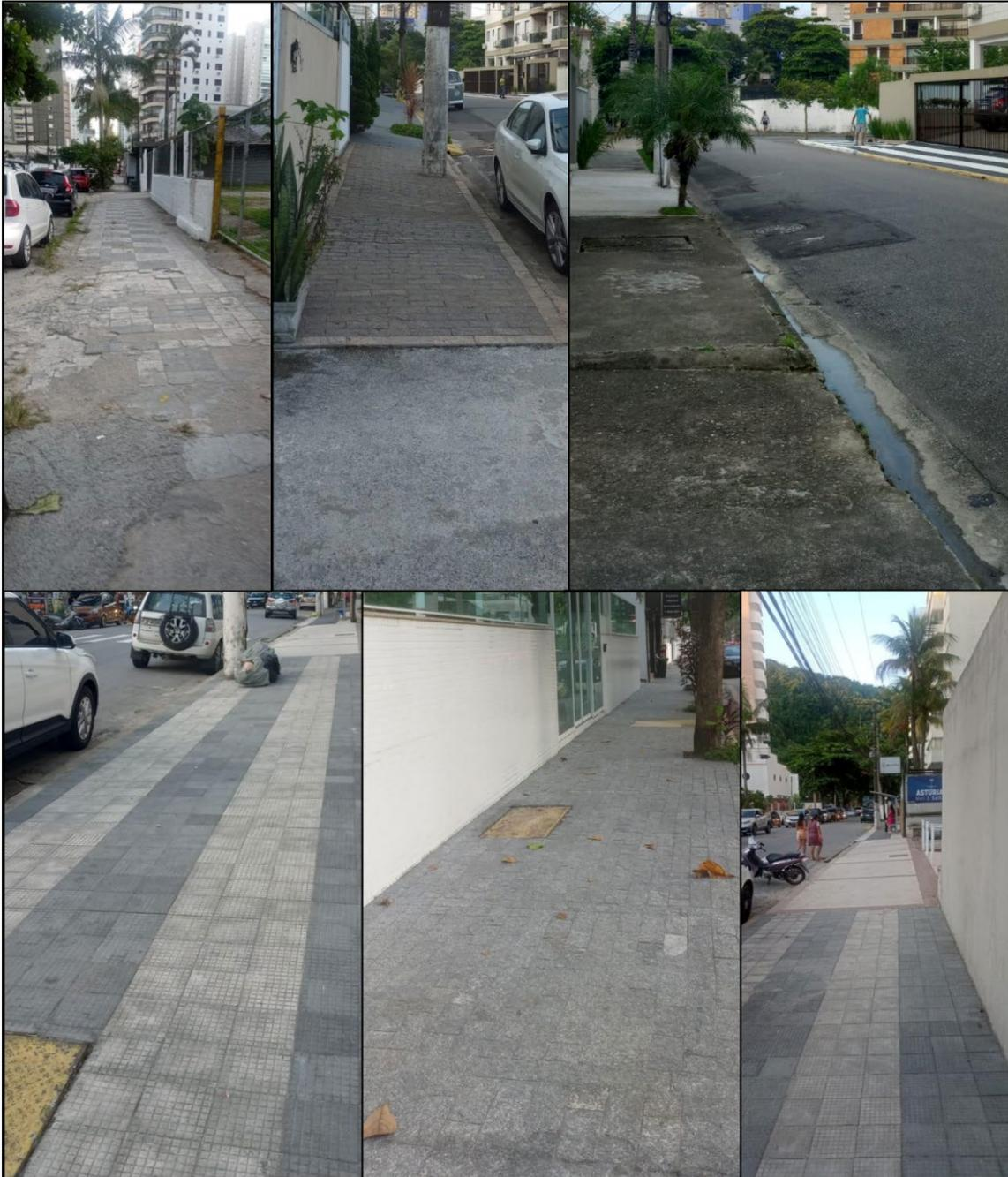
**Figure S8.** Uneven and/or drilled walkways of low-quality pavement of Guarujá city urban walkways.
